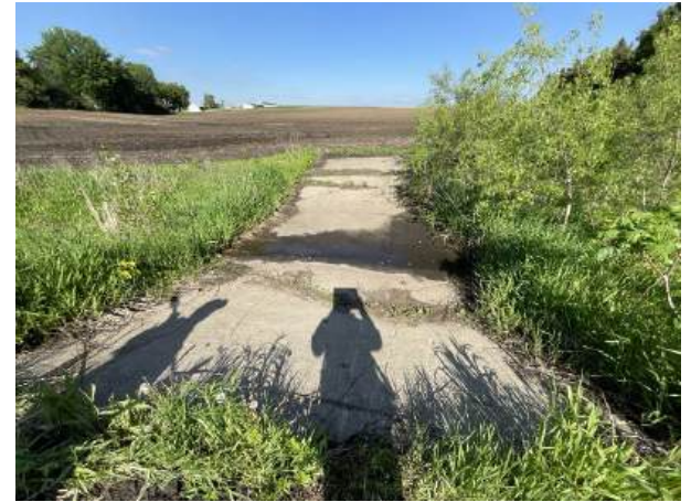
Photo 9: View of concrete structure between Wetland 2 and Wetland 3.
